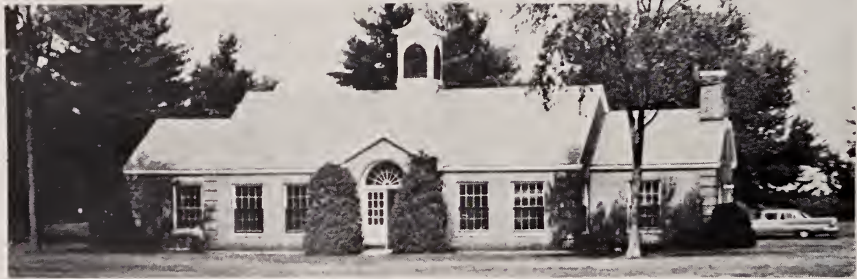
Brown's Crossing Pumping Station
